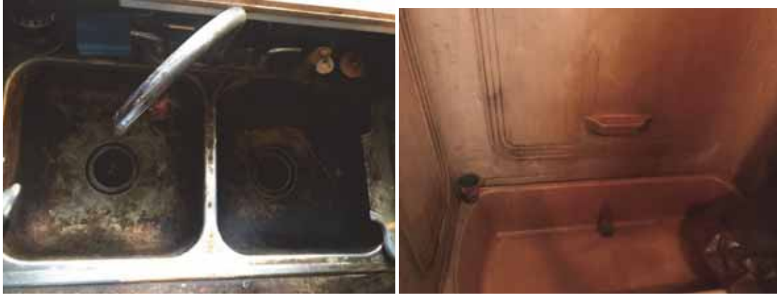
The kitchen sink and bathtub, discolored by iron and manganese in water, in a home near a mountaintop removal mine on Coal Mountain in Wyoming County, West Virginia © 2018 Human Rights Watch
