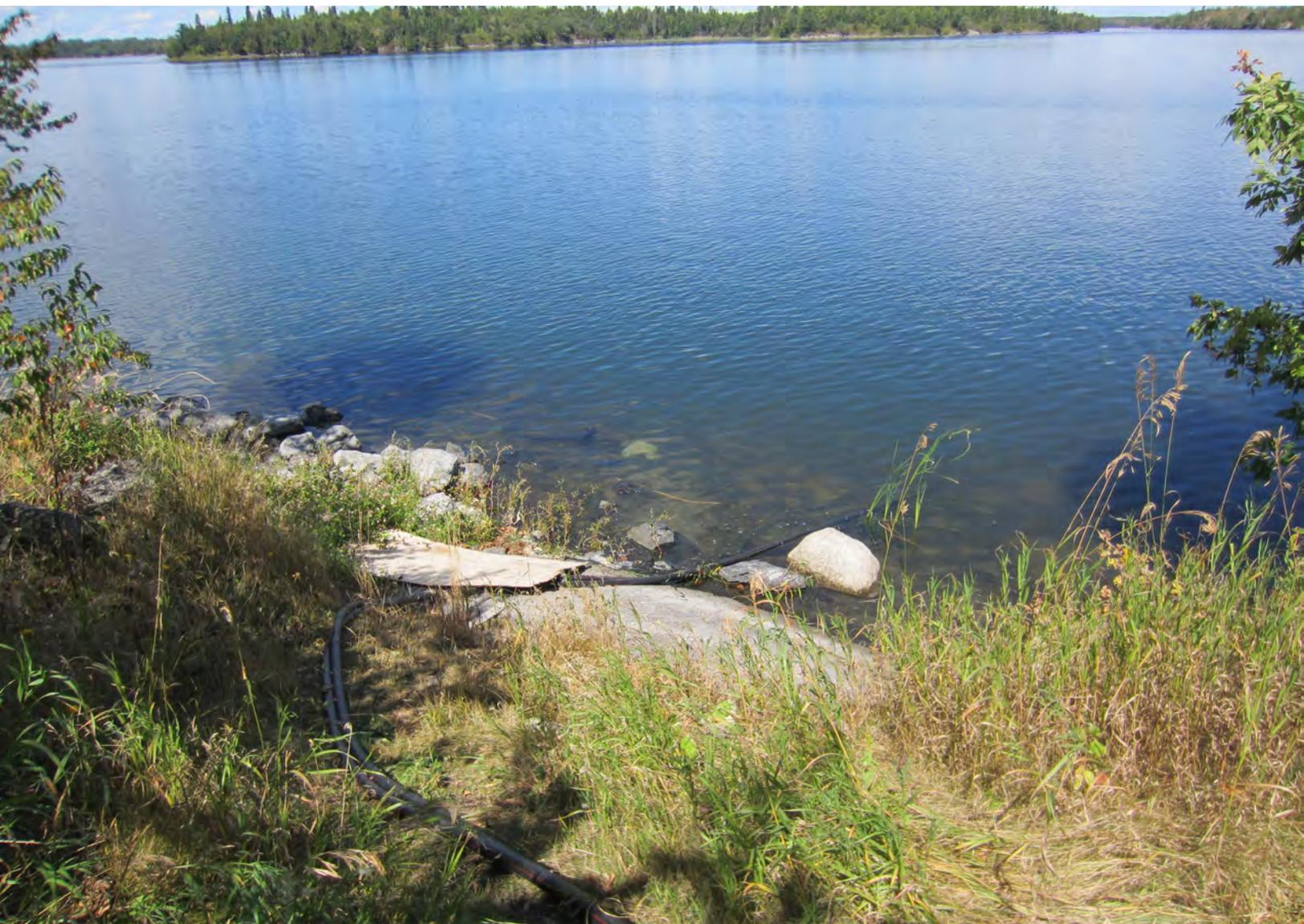
Pipe in Shoal Lake 40 First Nation which has been under a boil water advisory since 1997. The pipe delivers raw lake water to a pump house for disinfection, before it is pumped out to households for domestic use. © 2015 Amanda Klasing/Human Rights Watch
