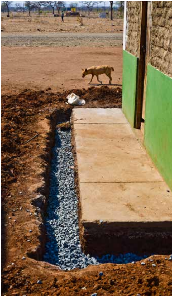
During the initial building phase, Vale changed the agreed-upon design of the new houses to a model with no foundation to hasten construction. Upon complaints by the resettled households, Vale began to repair all the houses in Cateme and 25 de Setembro in 2012, including by adding a foundation.
